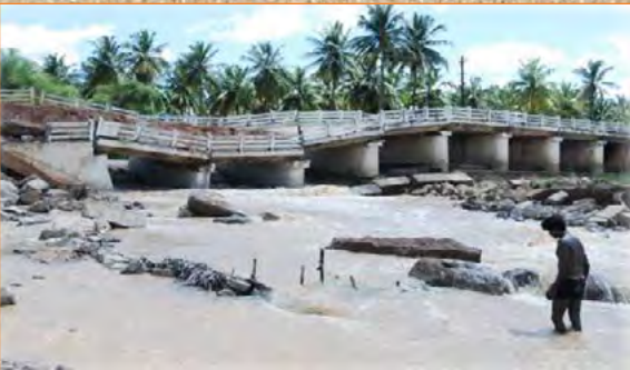
The Yaladabagi bridge in Sira taluk in Tumkur district which gave way because of sand mining. Photo: By Special Arrangement
