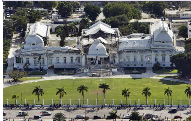
The Haitian Presidential Palace in Port-au-Prince, Haiti. Originally a two-story structure; the second story completely collapsed. Source: https://commons.wikimedia.org/wiki/File:Haitian_national_palace_earthquake-edit.jpg
