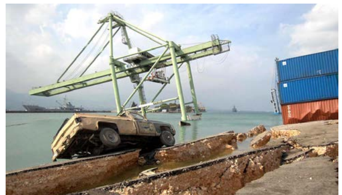
Port-au-Prince Harbour facilities, collapsed crane. Source: https://upload.wikimedia.org/wikipedia/commons/b/b7/Port-au-Prince_harbour_crane_after_2010_earthquake.jpg
