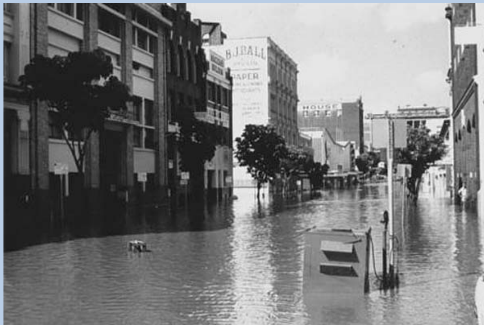
A flooded Charlotte Street in Brisbane's CBD, January 1974.
