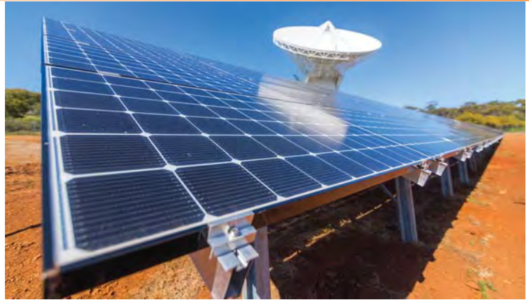
ESA's deep-space ground station at New Norcia, Western Australia, is now powered in part by sunlight, from a new solar power 'farm' completed in August 2017. The farm has 840 photovoltaic panels arranged in five double rows with a rated capacity of 250 kW. Source: https://commons.wikimedia.org/wiki/File:New_Norcia_solar_ESA387214.jpg
